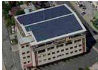
Installing solar PV system, PCKK, Palau Maldives
